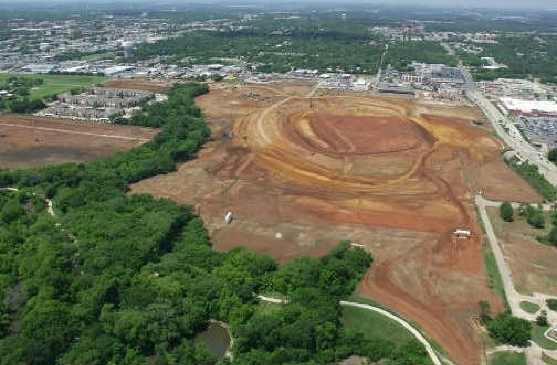
Cowboy Stadium Construction - May 4, 2006
