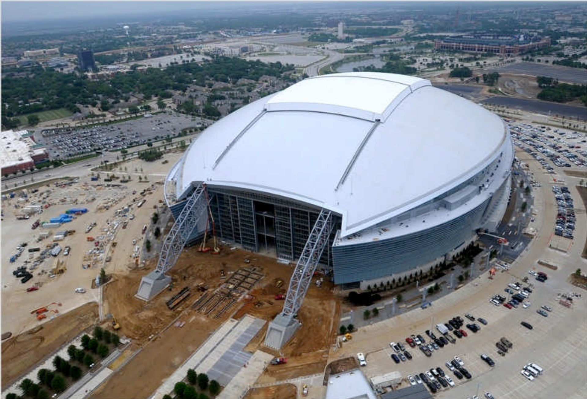
Cowboy Stadium Construction – May 1, 2009
